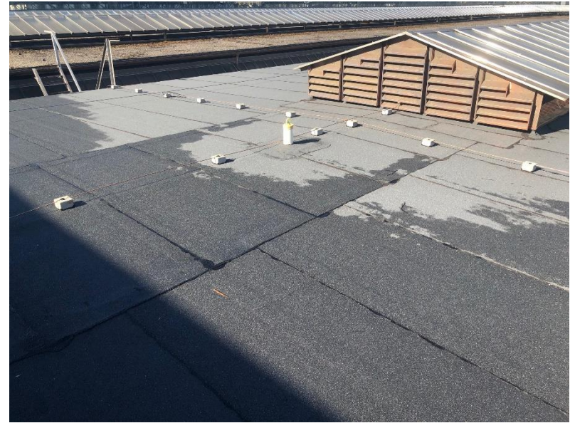
Finished roof incl. lifeline and lightning rod
