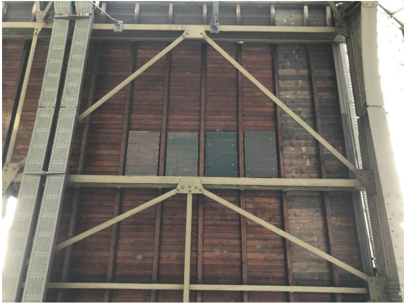
Color test array for replaced timber
